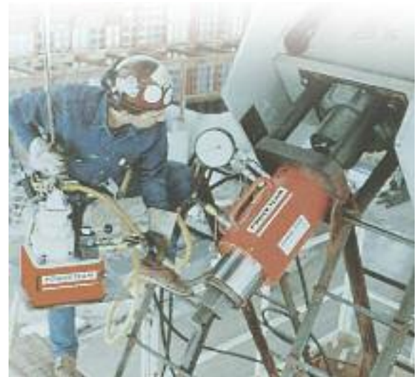
PA554 pump and RH2008 Center Hole cylinder used to tension cables.
